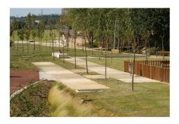
**Urban Park in the Perelló area, by Ruisànchez Architects. Vilablareix, Girona (Spain)**The park was devised to be a system of alluvial terraces, arranged in parallel to the river Güell to enable an increase in the capacity of the water course with avenues of water. The park conserves abundant riverside vegetation. The project's social success is, without doubt, its best endorsement.
